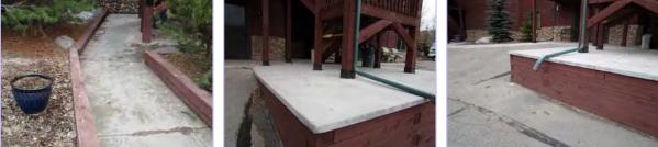
The tie planter boxes and retaining walls are in overall good to condition with some signs of deteriorated wood and minor movement, particularly at building 1. It is anticipate that the wood at building 1 will be repaired in conjunction with the concrete replacement project. Anticipate replacing areas as needed. Areas where ties are used as steps should be monitored closely and any trip and fall hazards should be repaired immediately.
